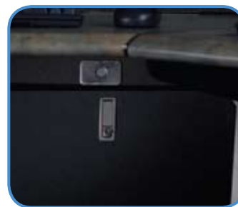
Additional cable grommets located beneath worksurfaces
