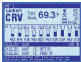
Bar graphs show the inlet temperature of every rack with a 2T temperature sensor.
