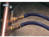
Liebert XDR-W modules are connected via quick-connect couplings to a Liebert XDP-W that controls coolant flow temperature and acts as an interface with your building's chilled water system through a heat exchanger.
