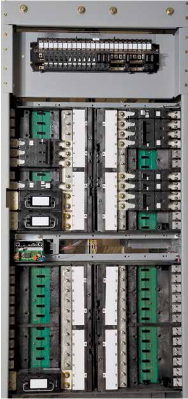
Distribution Bay with Fuses and Breakers Installed
