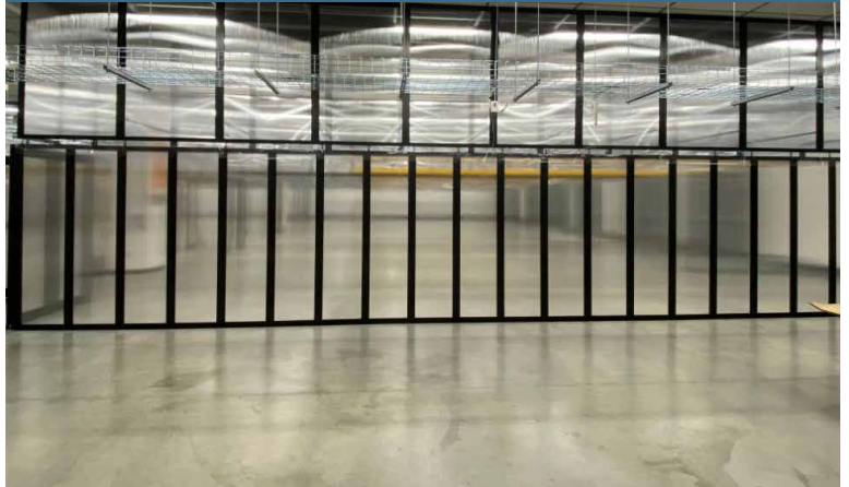
AISLE CONTAINMENT CEILING PANELS
