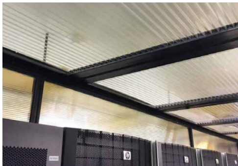
AISLE CONTAINMENT CEILING PANELS
